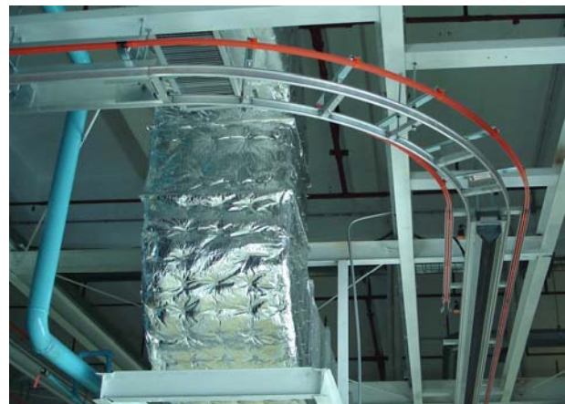
Return Rail - Bend with Bus Bar
